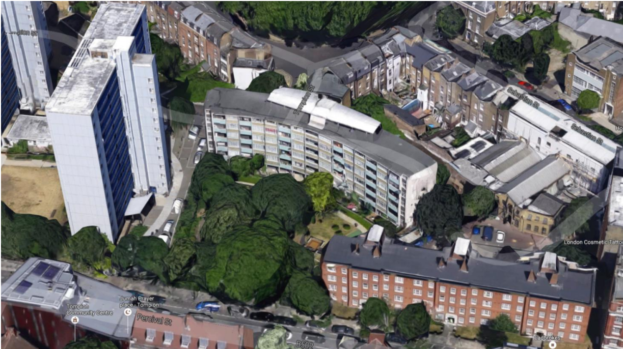
Image 2: Looking into the site in a Northerly direction
