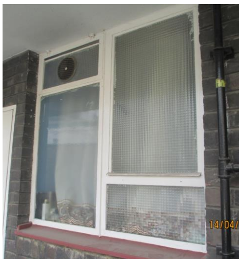
Image 7: Close up view of window style W14
