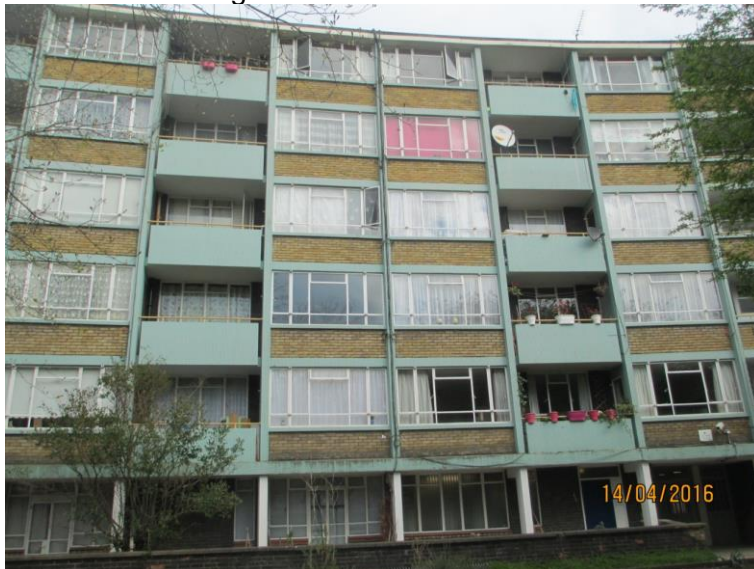
Image 6: View of rear elevation
